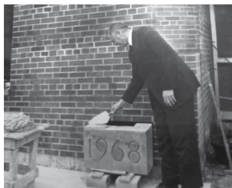
Board President Robert Nagowski smooths mortar onto bricks on the cornerstone of the brand new school at dedication ceremonies in May 1969.
